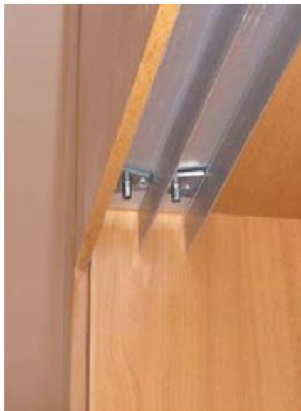
SLIDE SYSTEM OMEGA TOP RAIL DETAIL.
