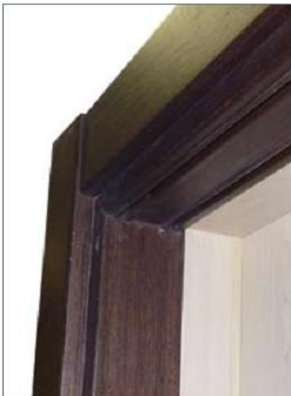
SLIDE SYSTEM TOP RAIL DETAIL.
