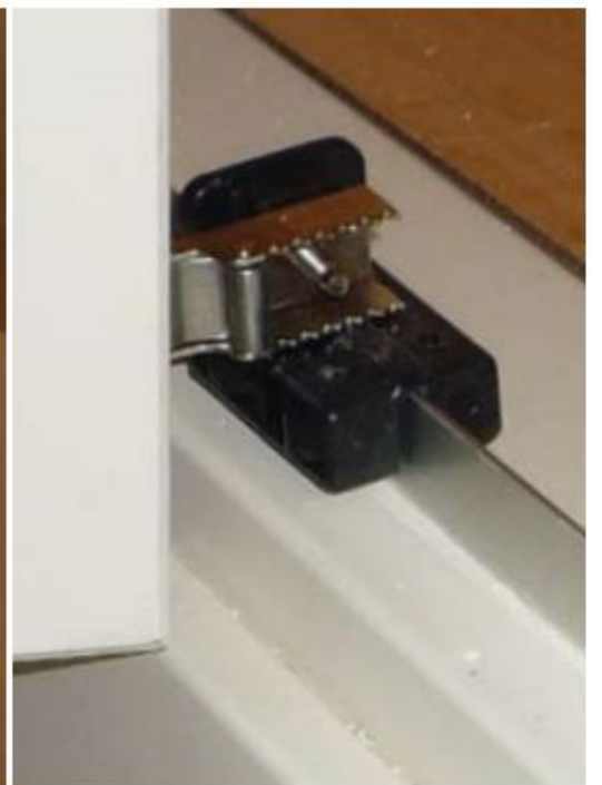
BOTTOM IRON FITTINGS FOLDABLE CUPBOARD DETAIL.
