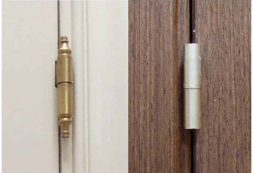
TRADITIONAL HINGE WITH ORNAMENTAL TIPS. TRADITIONAL HINGE WITHOUT ORNAMENTAL TIPS.
